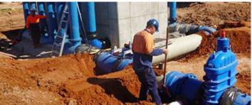
It modernised the irrigation systems across the Mildura, Red Cliffs and Merbein irrigation districts by replacing sections of channels with pipelines and upgrading pump stations to meet modern irrigation practices with a total cost of \$120 million. Clover was contracted to manufacture, supply and deliver over 20 kilometres of Superlit GRP, PVCO, Polyethylene and mild steel pipe and fittings in sizes up to DN2000 totalling over 6000 individual pipes and fittings and accessories.
