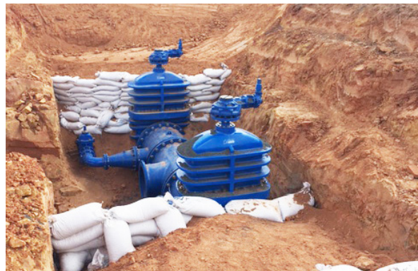
Gate valve assembly installation.
