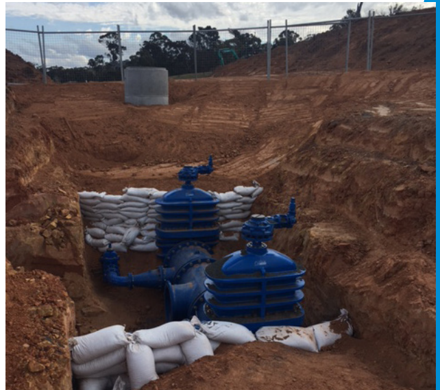
Gate valve assembly installation.
