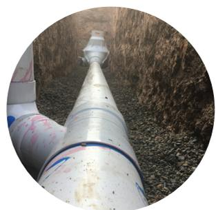
The PVC Maintenance Shaft is designed for access within a wastewater application, and the pipe geometry ensures good flow characteristics. The base design includes a sculpted channel to help direct flow, with 2 stage grade to assist with outflow. The outlet neck of the product is designed to cater for connections to larger maintenance equipment and allows for easier passing of rodding and CCTV equipment.
