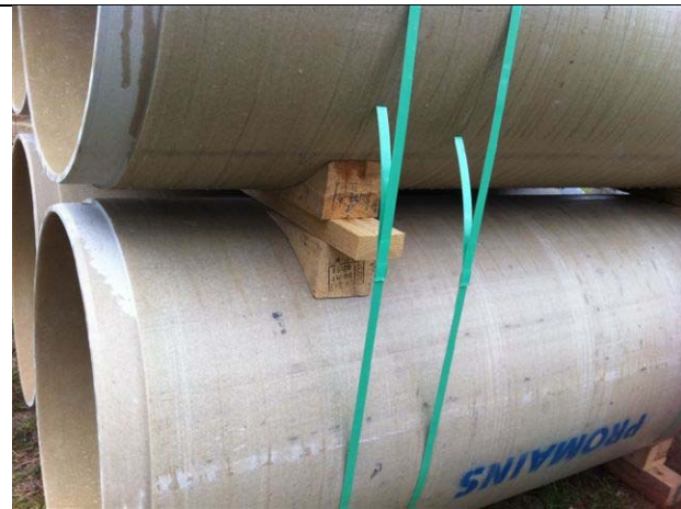
Photo 1 Storage of GRP CC- jacking Pipes
