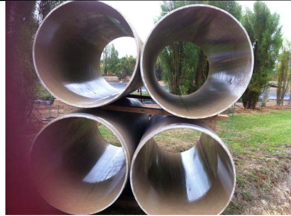
Photo 1 Storage of GRP CC- jacking Pipes
