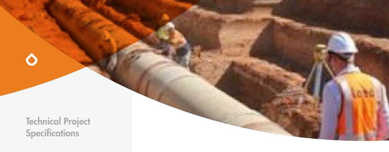
13,000m x DN2000 to DN300 Superlit GRP pipe and fittings.
